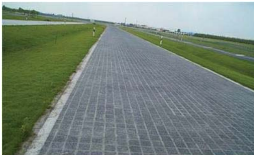
Figure 9. Belgian pavement.
